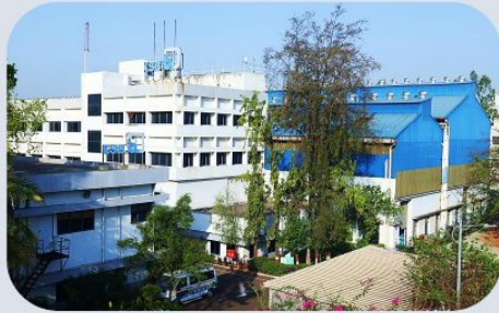
Dedicated spares manufacturing plant
